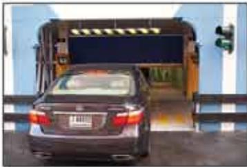
2. Drive into one of the convenient parking terminals indicated by a green light. Multiple automatic sensors ensure that the car is properly positioned for parking. Robotic Parking Systems offer more safety and security.
